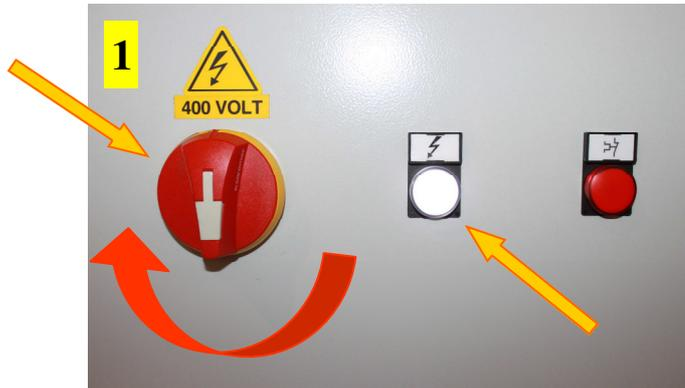
1) Rotate the main switch located on the switchgear. The white led should turn on.
